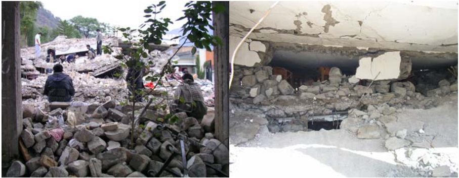
Fig. 1. Pakistan earthquake 2005, locals attempting to search for survivors in a collapsed girl's college. The structure was in unstable condition; excavation and lifting machineries were prohibited from the site. (Pictures taken on site by author during mission)
